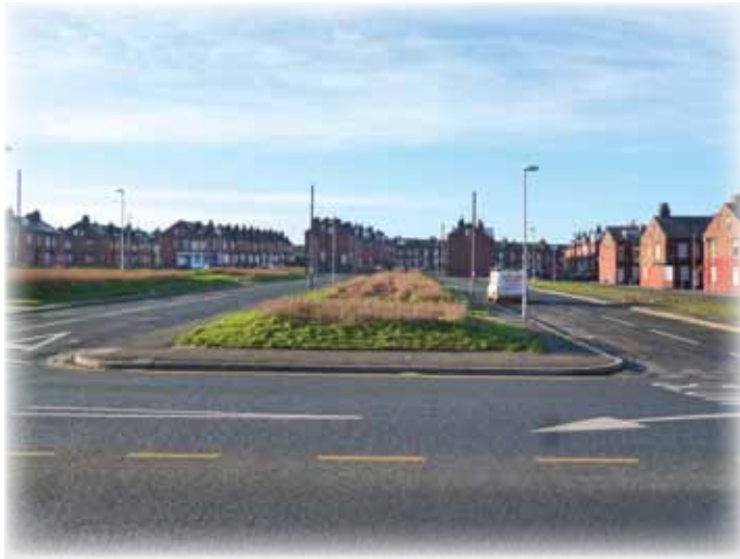
Above: Brown Lane East prior to any development.
