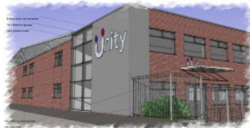
Work is set to start on the whole scale refurbishment of two of our enterprise centres. Works will include recladding roofs, new doors & windows, new lifts, PV panels, re-wiring, new signage and data cabling for faster broadband.
